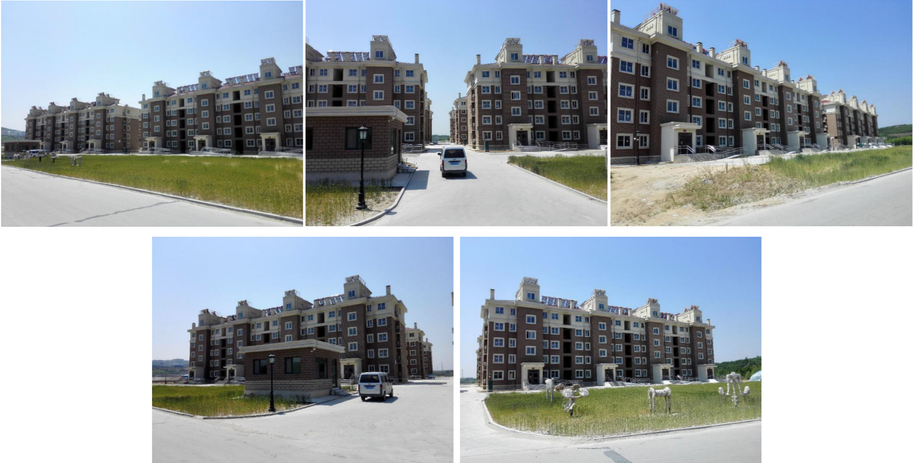
construction of housing for 280 families
