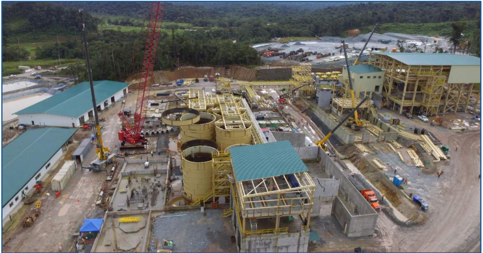
Aerial view of the process plant
