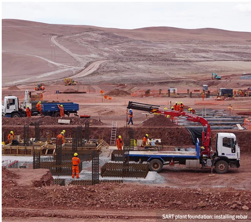
SART plant: installing rebar
