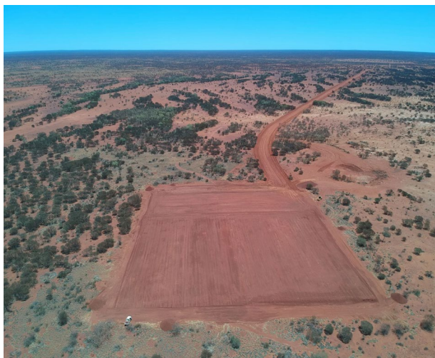
Clearing for the accommodation village
