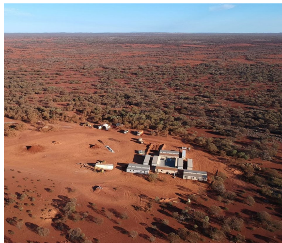
Installation of the construction camp
