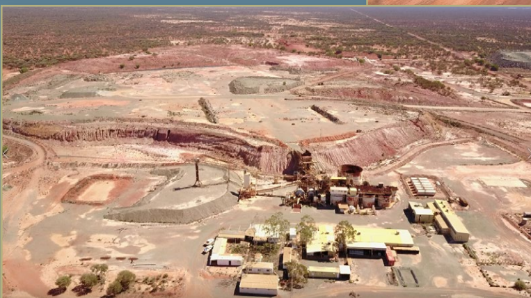
Extensive Site Infrastructure including 600,000tpa processing plant
