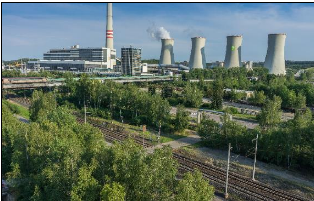
Photo 6-3: Current Power Plant
