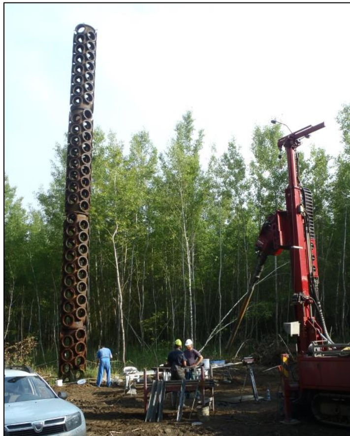
Photo 6-4: Historical Decantation Tower Located on Cell #3, Near Drill Holes T3-310, 311 and-318
