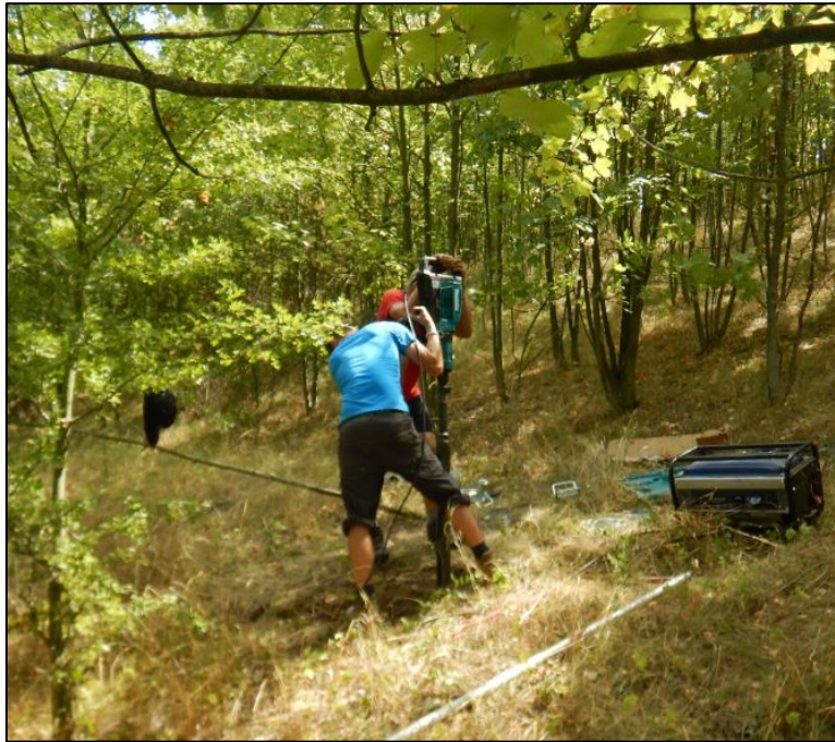
Photo 10-3: Drilling of Perimeter Embankment Hole using Hand Portage Percussion Drill
