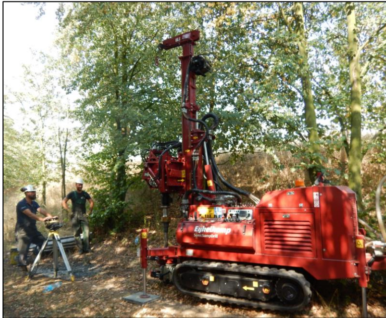
Photo 10-2: Eijkelkamp SonicSampDrill SRS Used for 2018 Sonic Drilling Investigation
