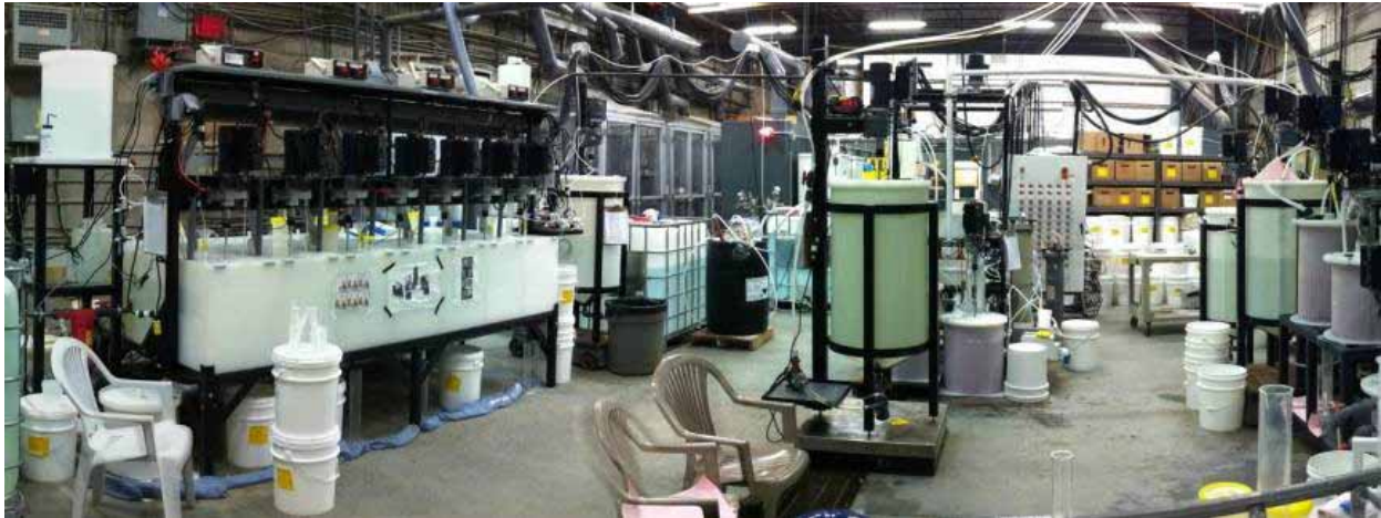
Figure 13.8 Pilot Plant (SX-Purification-Carbonation-Filtration-Washing Pulp)
