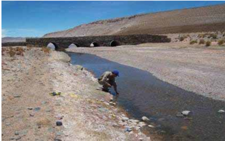
Figure 7.15 Rio Rosario Just Above the Highway 74 Bridge Crossing
